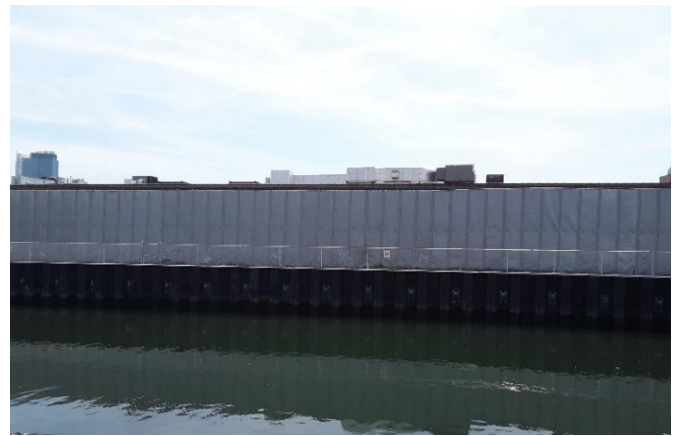
Completed Fulton MGP Sealed Bulkhead Barrier Wall Along Gowanus Canal.
